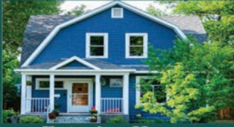
Exterior House Painting
