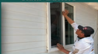
Custom Windows Installed
