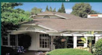
New Roof, Re-Roof, & Roof Repair
