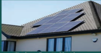
Solar Installation, Upgrade, & Repair
