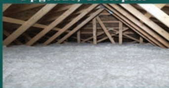
Attic and Wall Insulation
