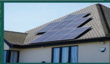
Solar Installation, Upgrade, & Repair
