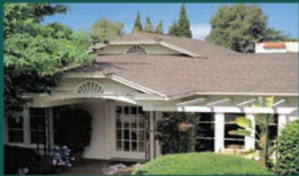
New Roof, Re-Roof, & Roof Repair
