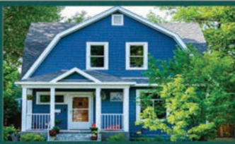
Exterior House Painting
