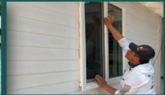
Custom Windows Installed
