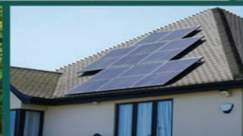
Solar Installation, Upgrade, & Repair
