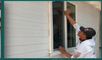
Custom Windows Installed
