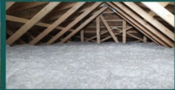
Attic and Wall Insulation
