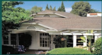
New Roof, Re-Roof, & Roof Repair
