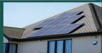
Solar Installation, Upgrade, & Repair
