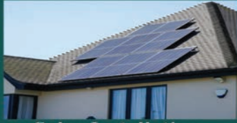
Solar Installation, Upgrade, & Repair
